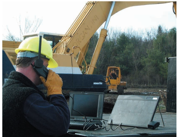
Project engineer on job site using the Portable Energy System
